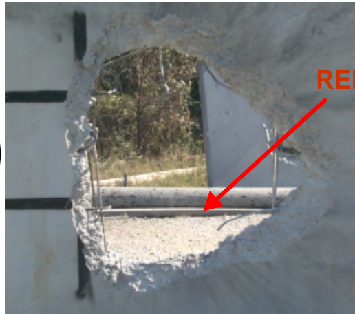
Rebar Hole Opening 34.5" x 34" Rebar on top could be bent 34.5" x 44" opening
