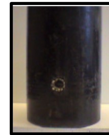
Full Penetration at Entrance Point
