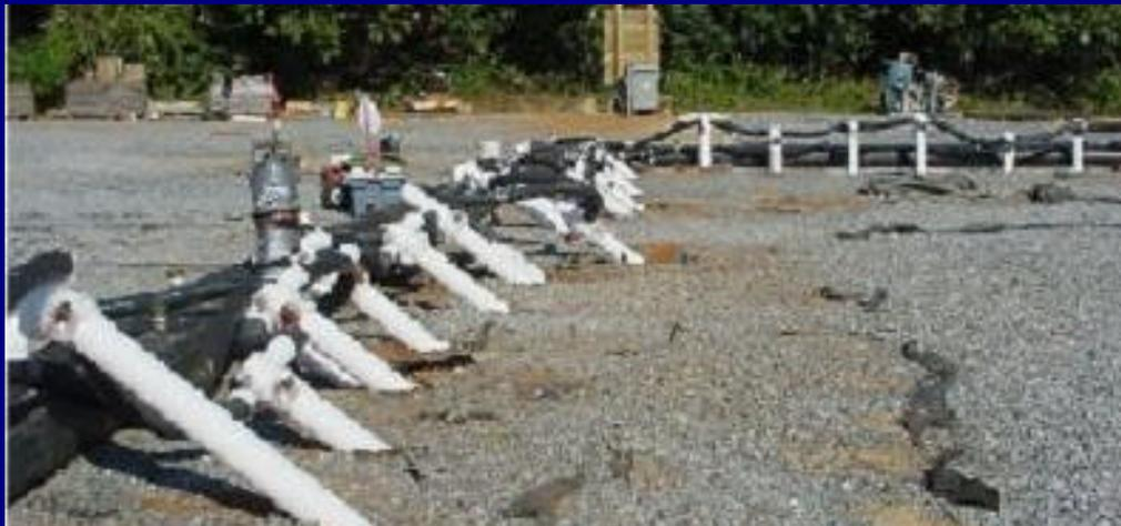
Installed Freeze Pipes (note frost on pipes)
