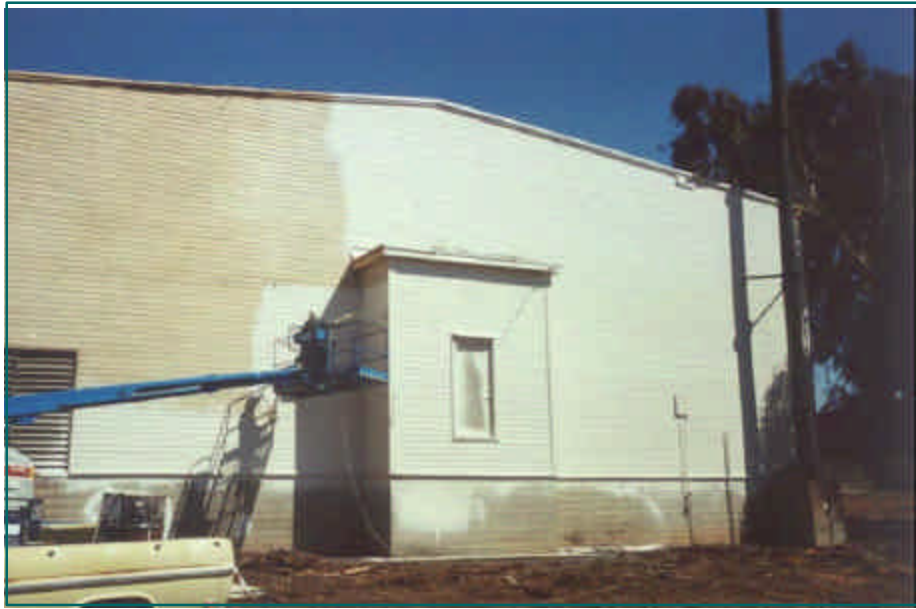
Application of EcoBond™
