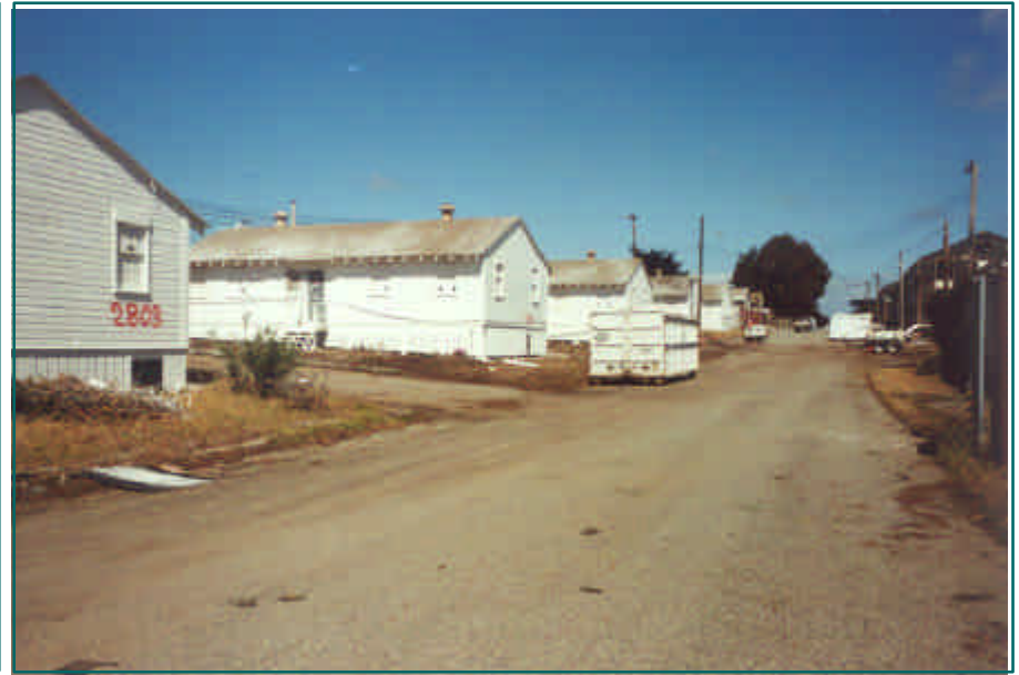
EcoBond™ coated buildings (awaiting demolition)
