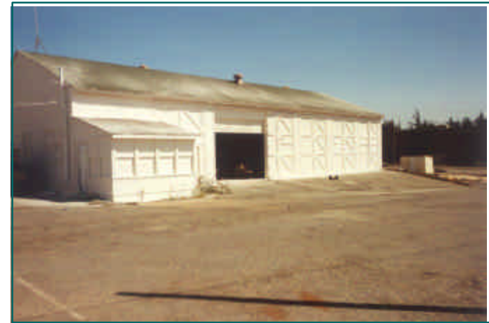
EcoBond™ coated building (awaiting demolition)
