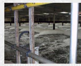
Data from REDMAP, combined with ongoing pollution prevention efforts, are enabling plant operators to optimize the biological treatment activity to reduce the amount of toxic sludge generated, which was reduced 60 percent in one year, despite wastewater volume increases.
