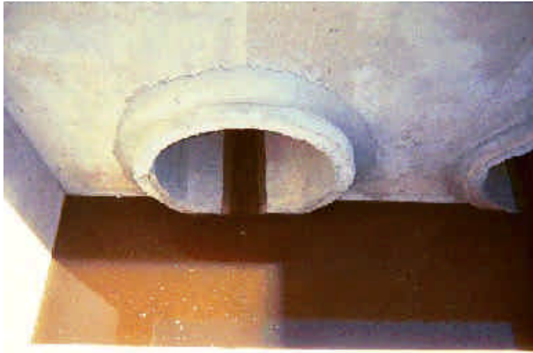
Outfall looking North.
