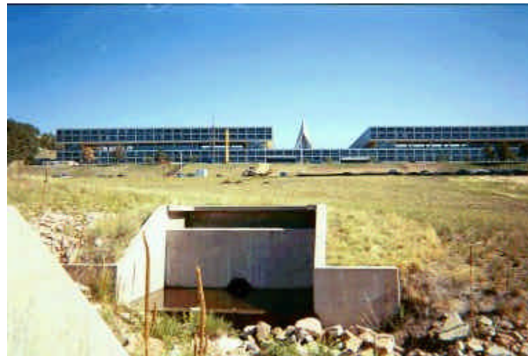
Outfall looking North.
