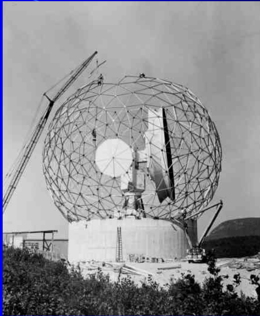
Construction of the A-Side Antenna in 1960.
