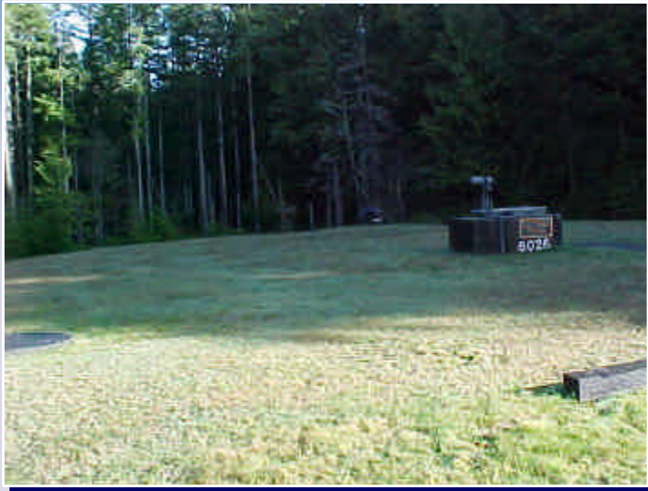
1,000,000 Gallon Water Storage Tank and Associated Piping
