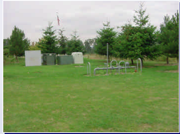
670 linear feet of Underground Electric and Natural Gas Lines
