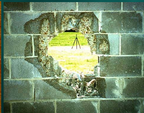
Concrete Wall (Exit)
