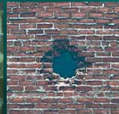
Brick Wall (Exit)
