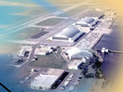
Communications Area Master Station
