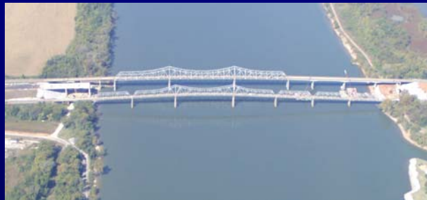
Whitesburg Bridge, HSV
