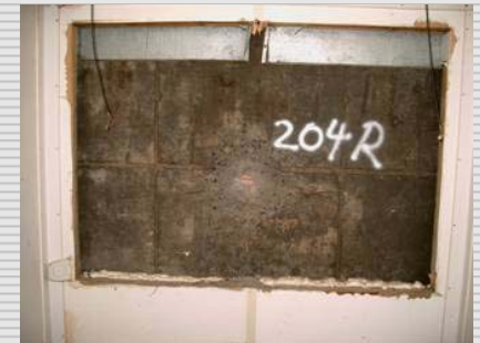
Rear side of concrete inside the container
