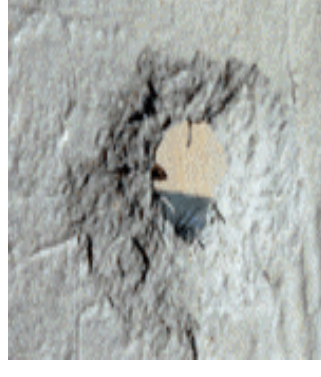
Double reinforced concrete wall
