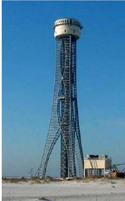
Fig. 6: Santa Rosa Island Open-Air Hardware-in-the-Loop tower at Eglin site A13B.
