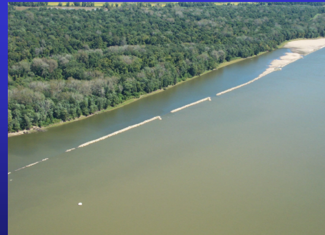
Notched Off-Bank Revetment
