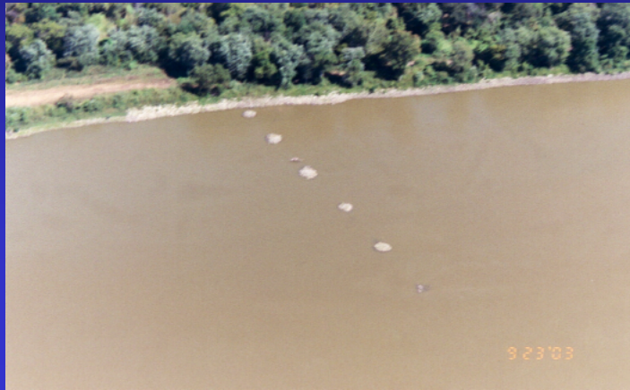
Multiple Round Point Structure
