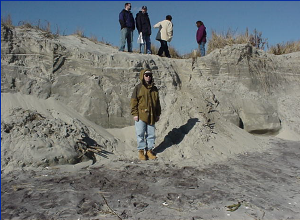
North End Closer to Inlet January 2003
