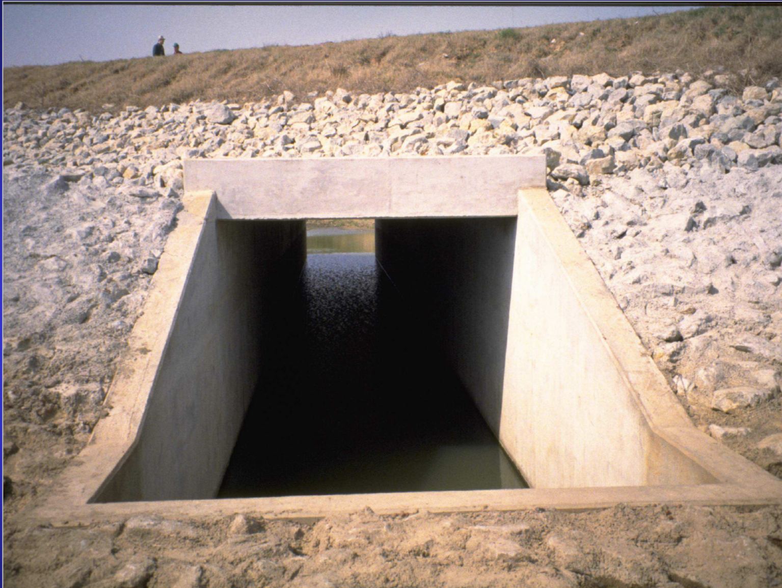
Box Culvert Grade Control Structure
