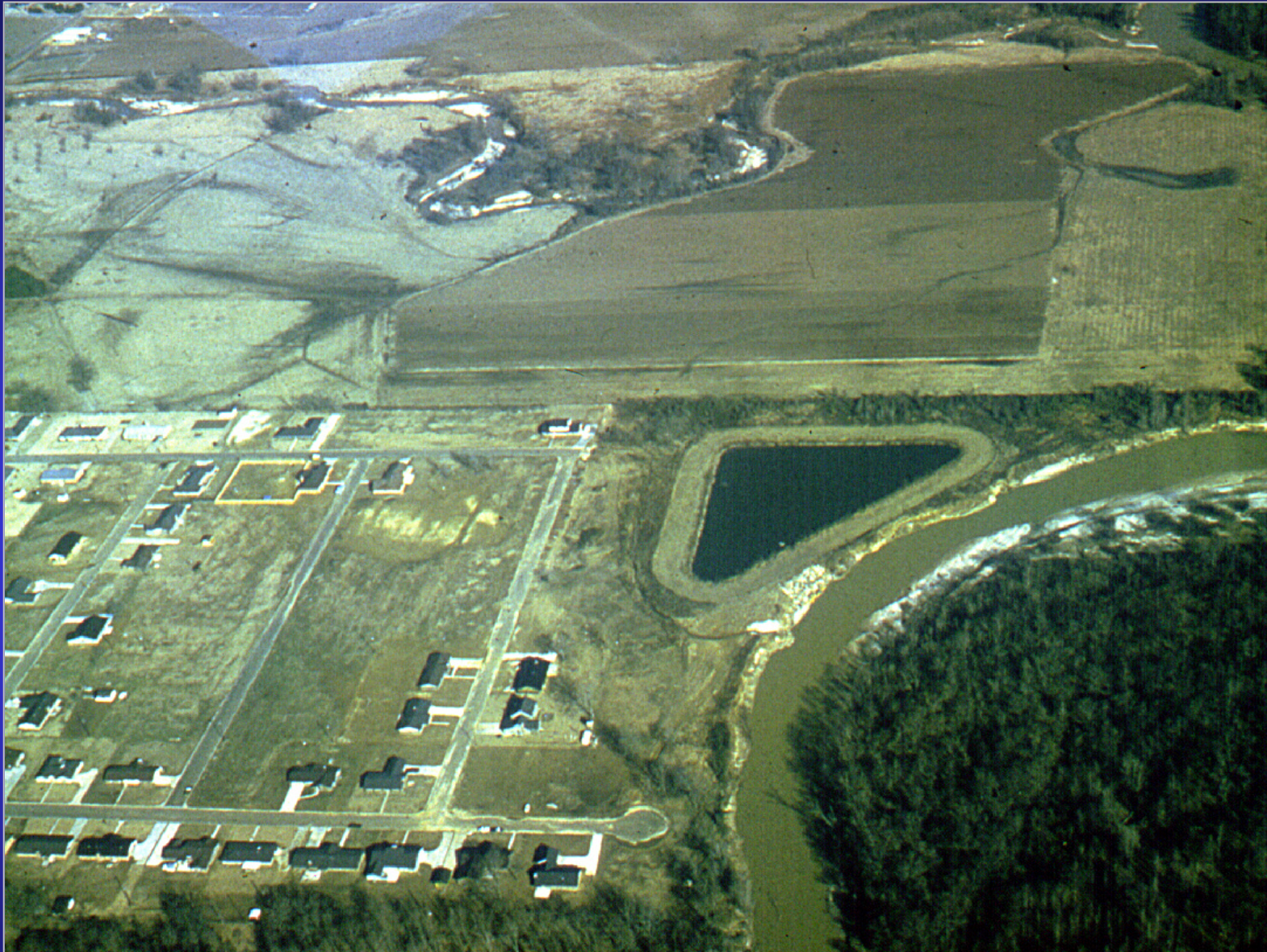
Effects of Bank Erosion
