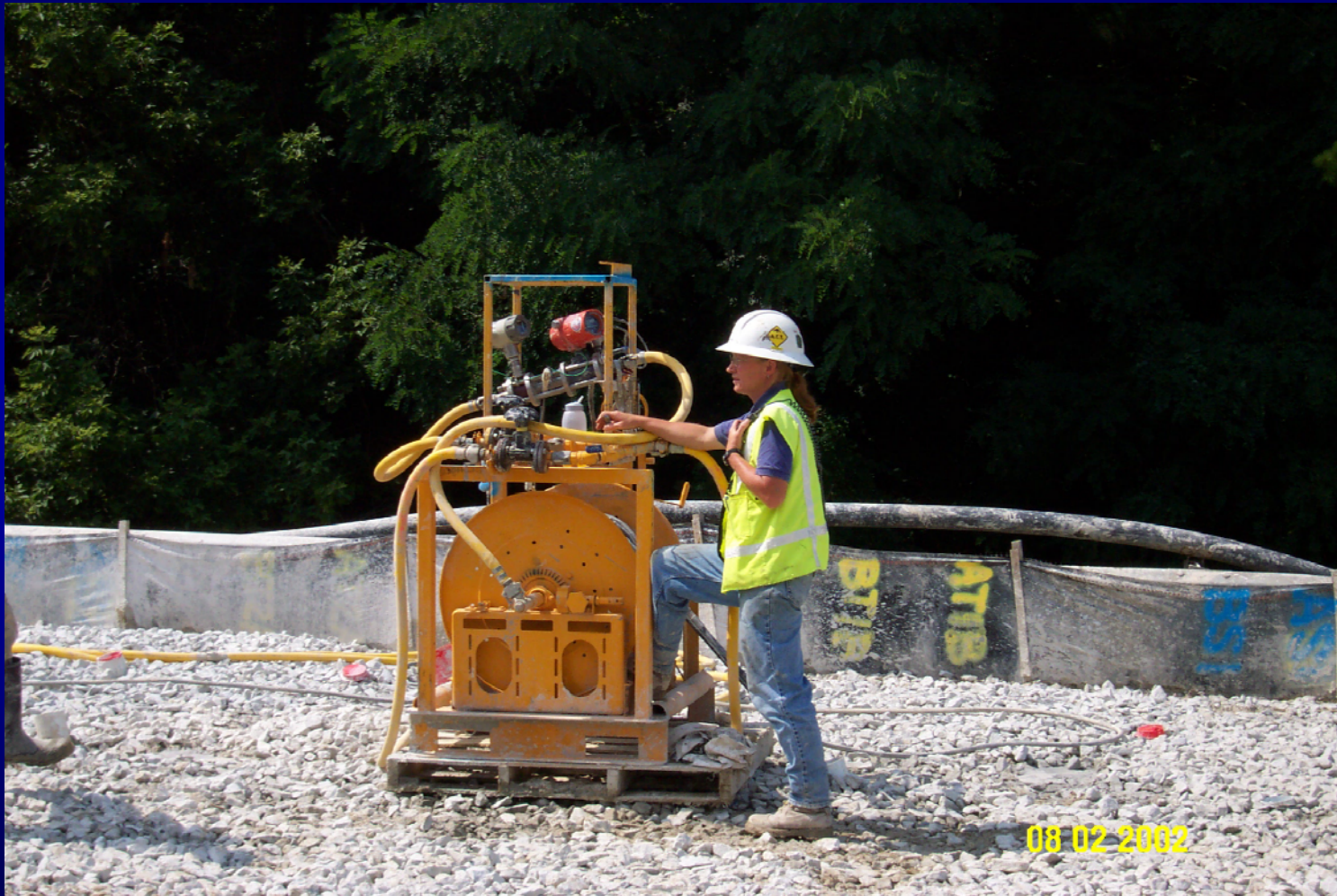
Grout Header Controls
