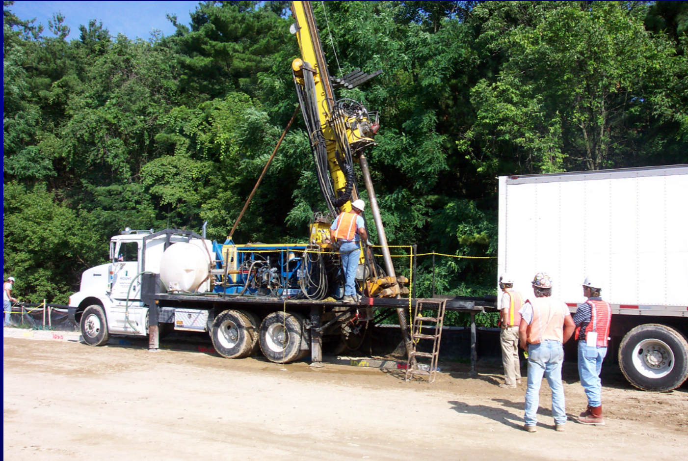
Rotosonic Drill Rig
