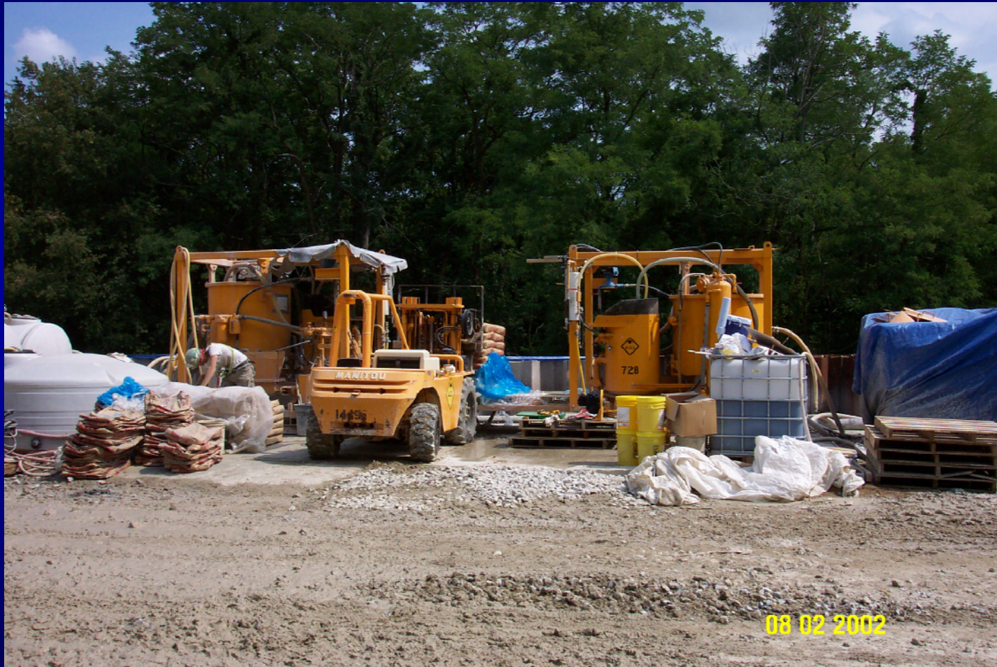
Two High Speed/High Volume Grout Plants
