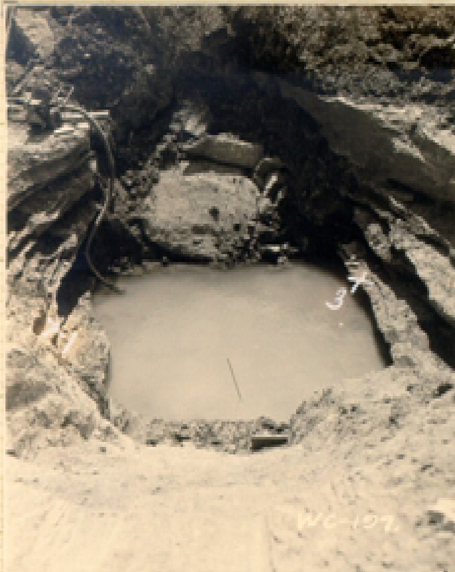
4-2-42. Looking SE along hole at trench sta. 27+95. IV-A
