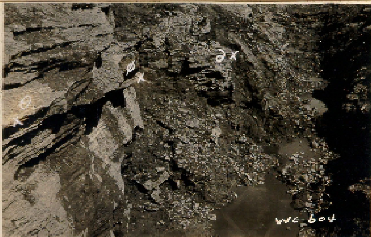
8-27-42. Looking SE in trench from sta. 5+50.
