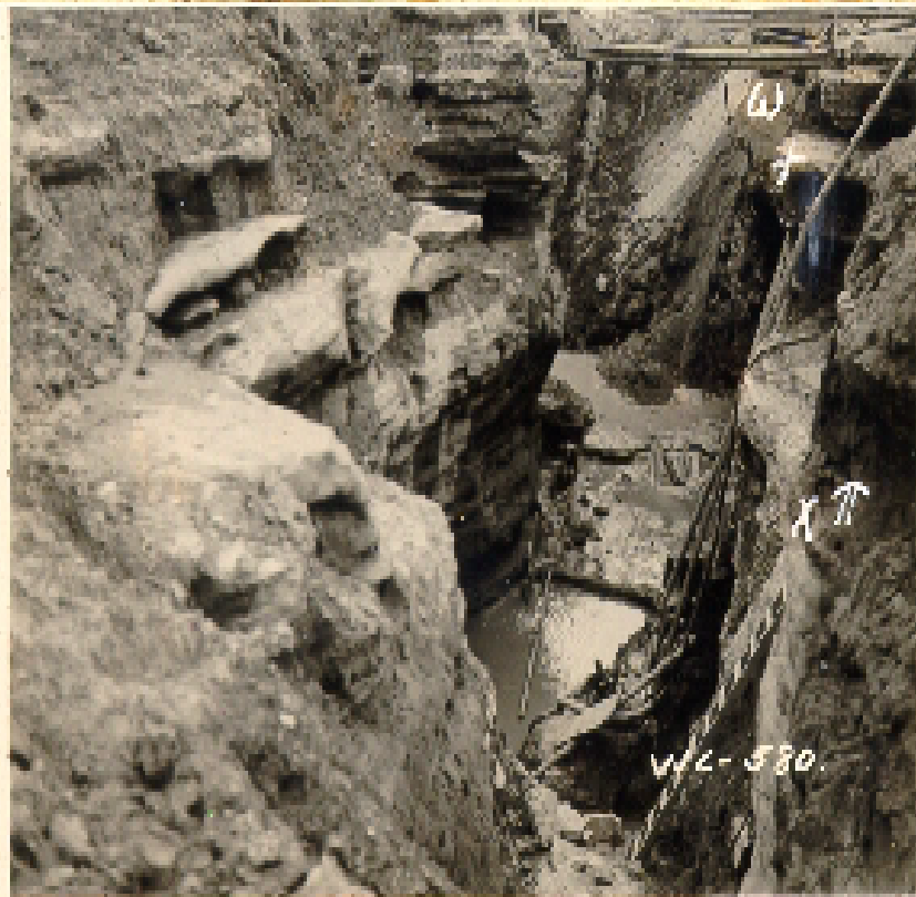
8-23-42/looking S in trench from vicinity embankment sta. 36+10. I-6
