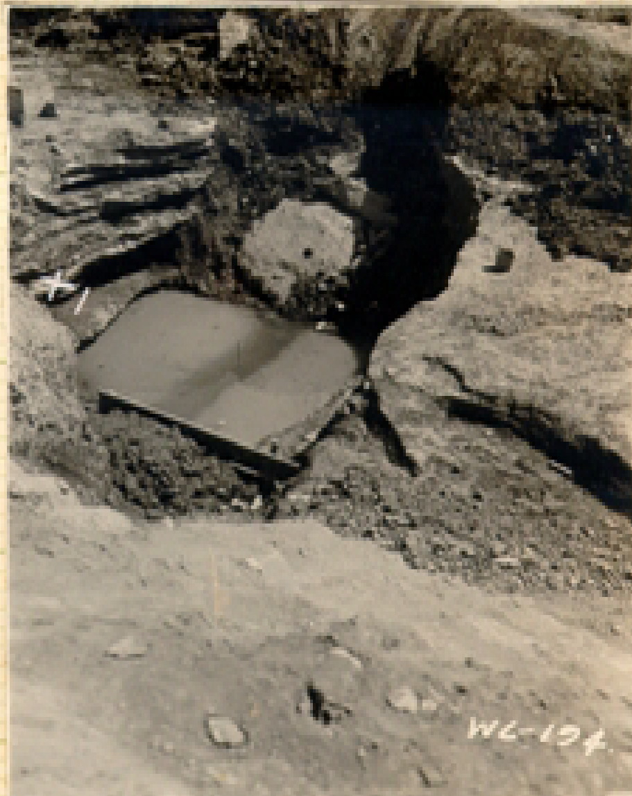
4-2-42. Looking E across hole at trench sta. 27+95. IV-B
