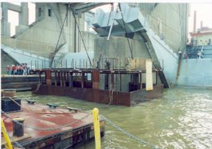
Temporary dewatering box built by LRS to make limited scour repairs around piers at the Markland Project.
