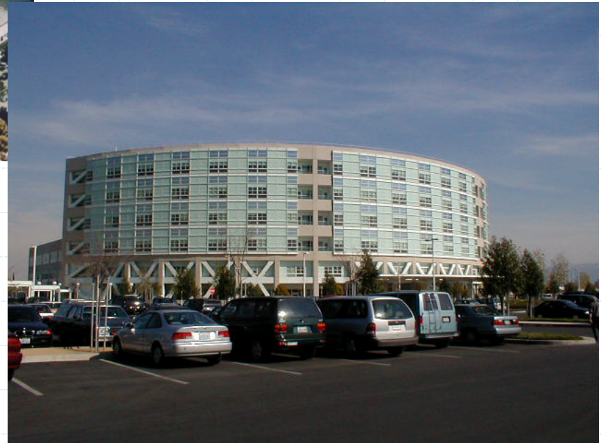
SAN BERNARDINO HOSPITAL, CA, ELASTOMERIC BEARINGS AND FLUID VISCOUS DAMPERS
