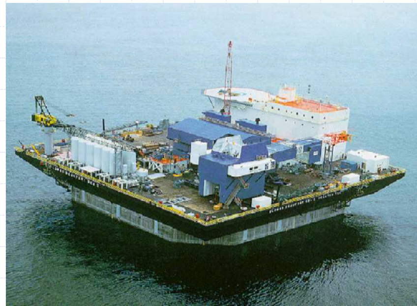
OFFSHORE GAS PLATFORM WITH CONCRETE GRAVITY BASE
