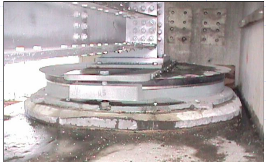
BENICIA-MARTINEZ BRIDGE SAN FRANCISCO BAY AREA FP BEARINGS
