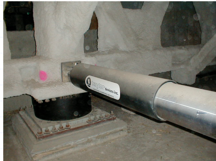
SAN BERNANDINO HOSPITAL, CA, ELASTOMERIC BEARINGS AND FLUID VISCOUS DAMPERS
