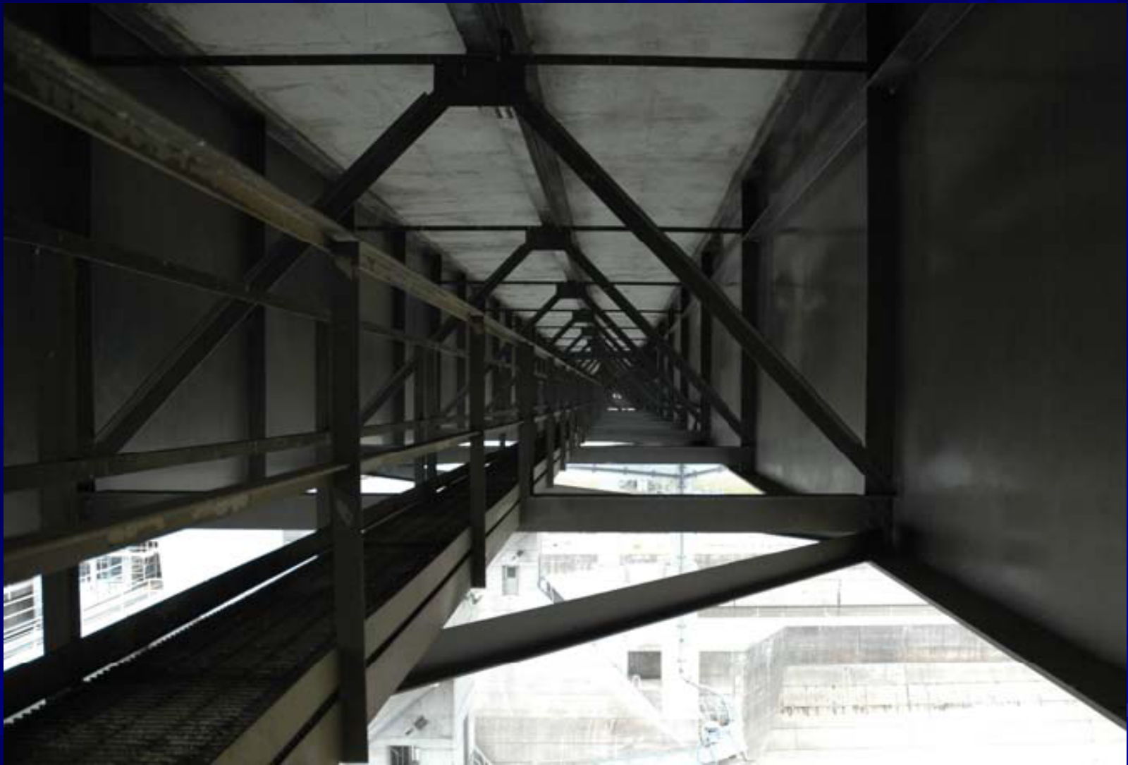
View of typical cross frame in Unit 1 (and Unit 3).
