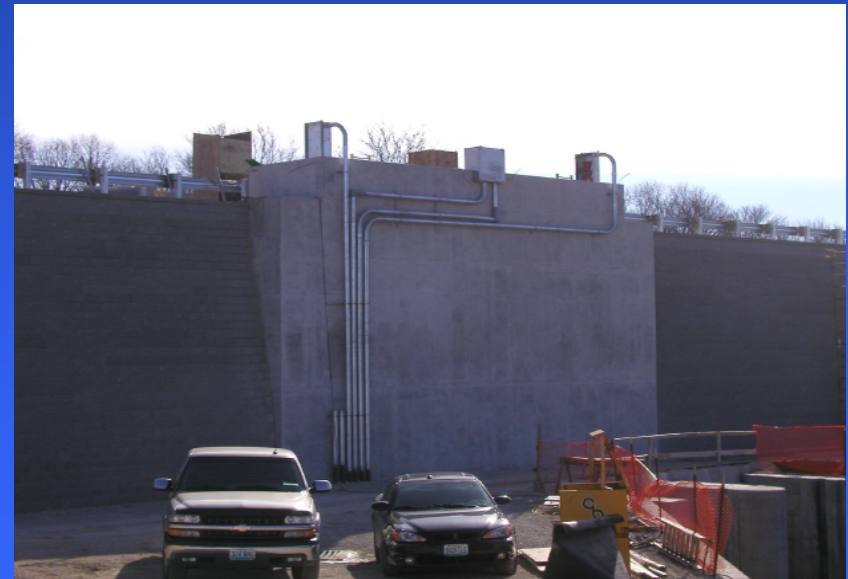
PUMP STATION WITH MSE WALL
