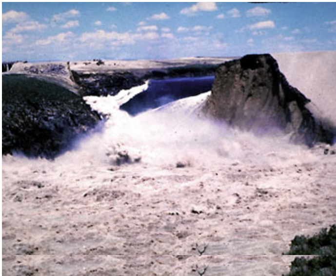
Teton Dam failure, ID, 1976
