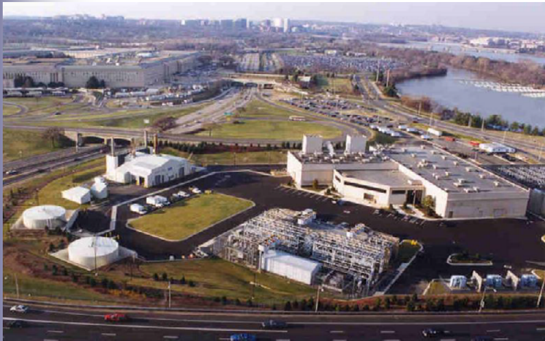
Heating & Refrigeration Plant (design & construction 1992-1997 )
