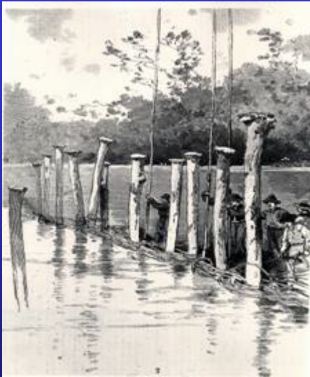
Workers Constructing Pile Dikes
