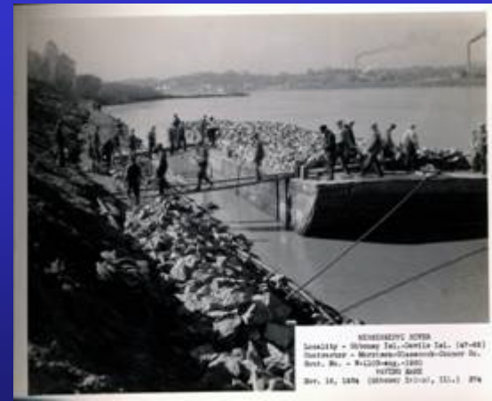
Hand Placing Stone Riprap
