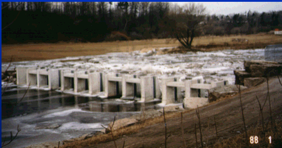
1986 Credit R., Mississauga, ONT., Piers 6-ft-apart, grounded jam in channel, bypass flow via floodplain.
