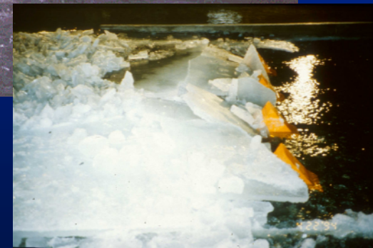
1994 Lamoille R., Hardwick, VT., Grounded jam behind boulders, 14-ft gaps, bypass flow via tree covered floodplain (CRREL design). Monitored by CRREL as field site. No ice jam flooding since construction.
