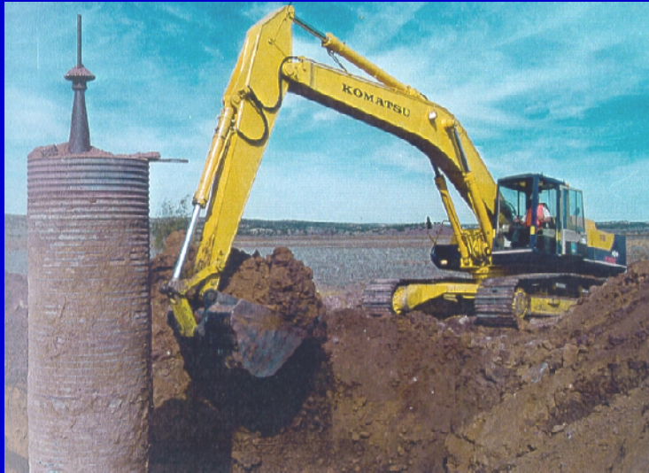
Excavation of the existing conduit
