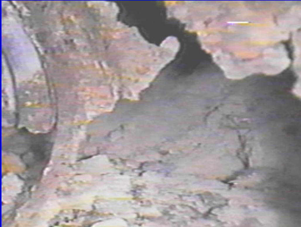
Corroded CMP
