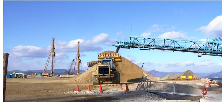
**Sand Piles: Liquefaction Prevention from Tight Consolidation
