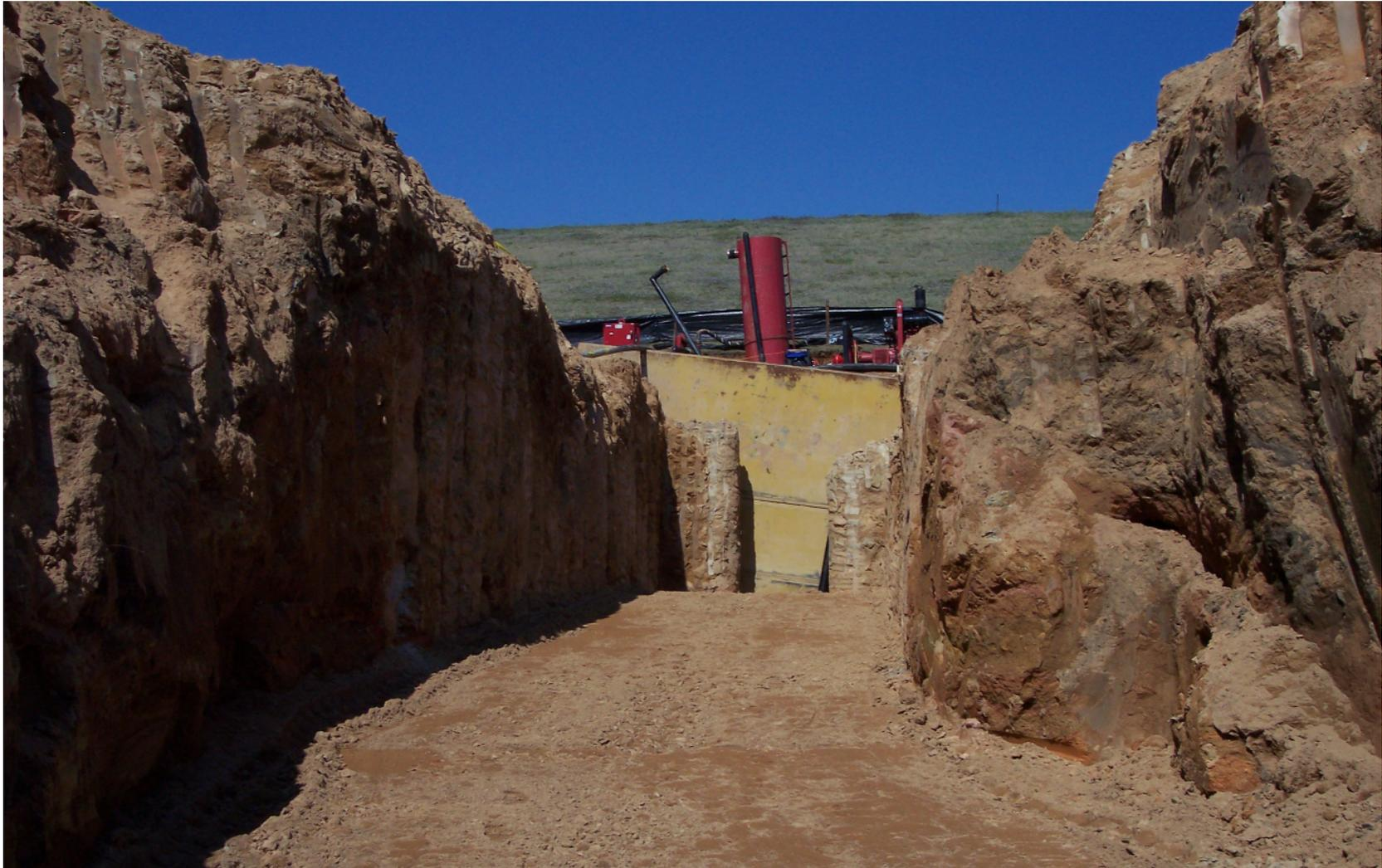
Installation of discharge line; note slot in longitudinal wall
