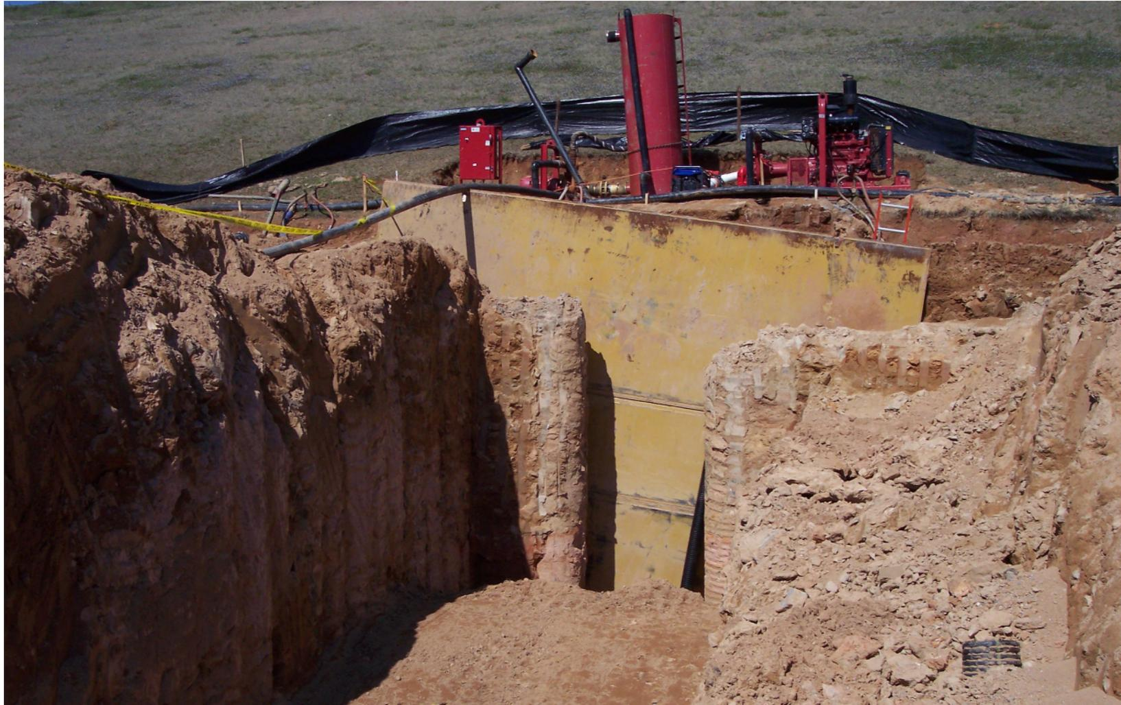
Trench box and dewatering pump station
