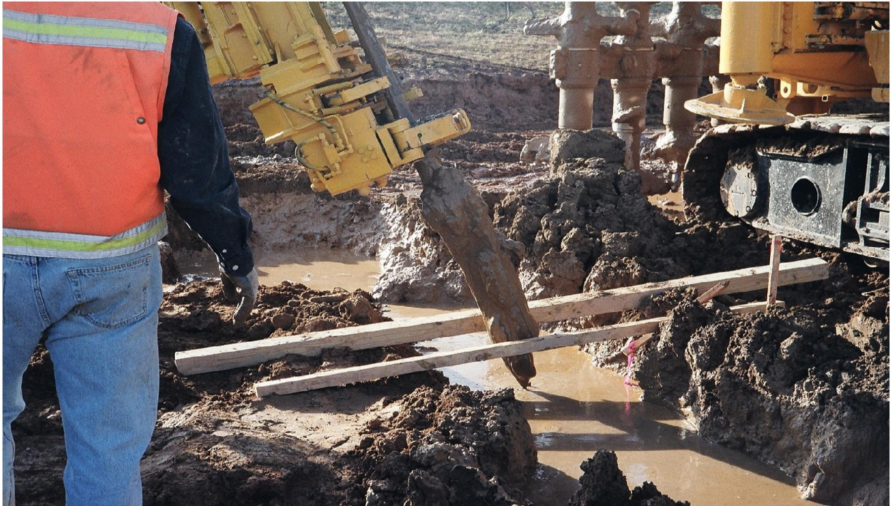
Sampler plugged with soil from unimproved zone
