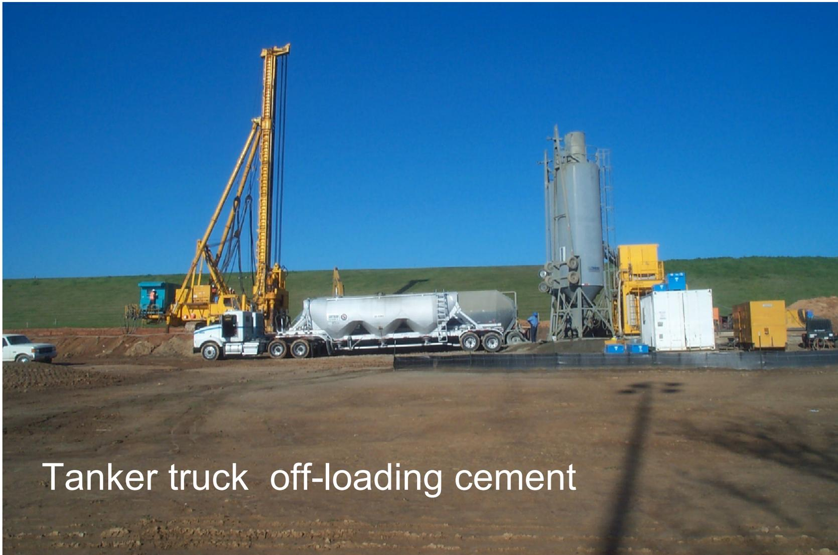
Tanker truck off-loading cement
