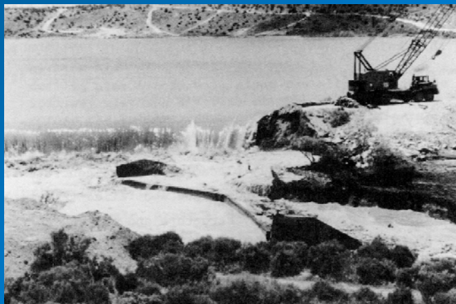
Spillway Breach
