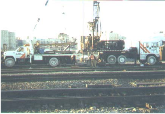
High-rail, turn-table mounted Sonic rigs
