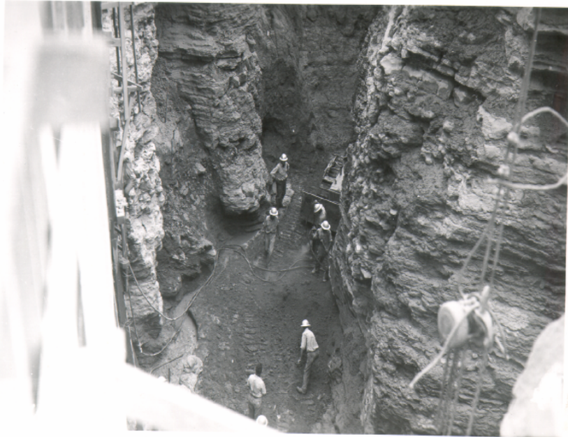
61/421 14 August 1947 Filling core trench, Mon. 37
