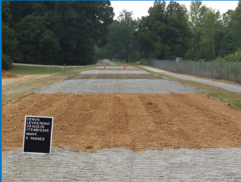
Maintenance Test Section
