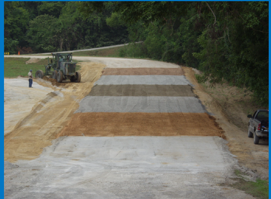
New Construction Test Section
