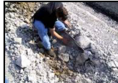
Test Pits – Verify Cracked Pattern
