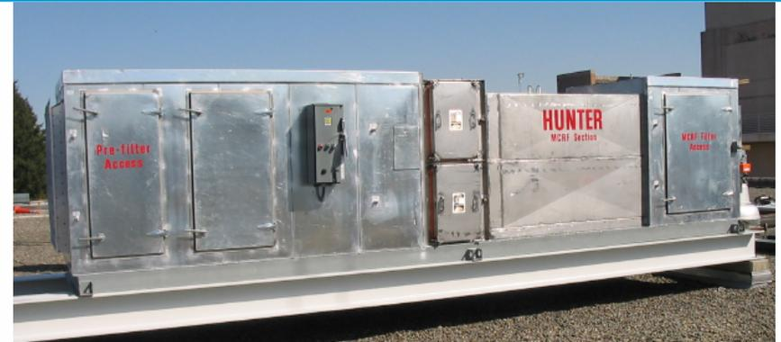
Multi Cell Radial Flow Filter Housing
