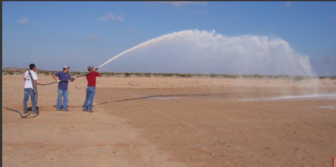
Isotron lockdown application with hydroseeder prevents personnel contact.
