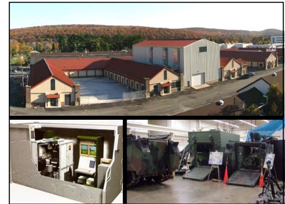
Armament Technology Facility
