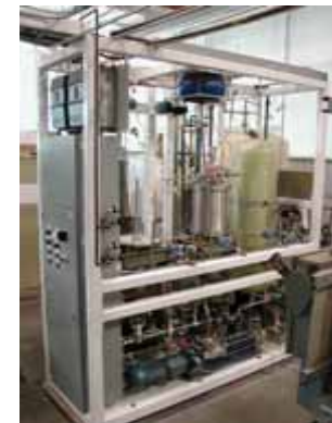
Heavy Metals Removal
