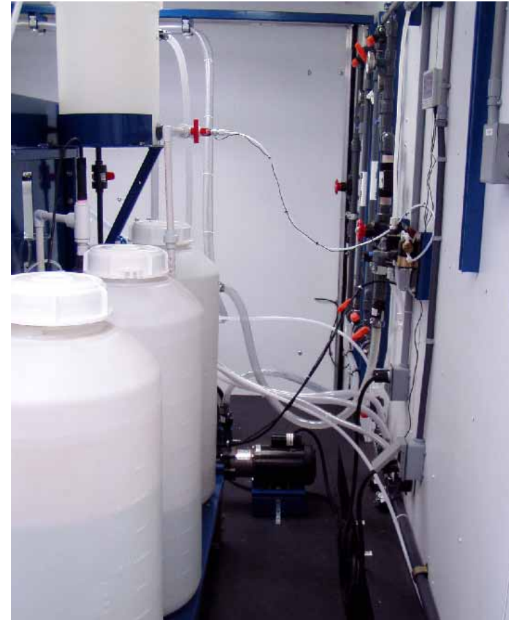
Pilot Reactors and Membrane
