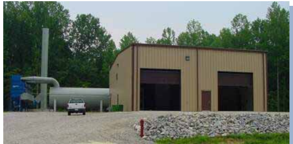
D-200 CDC Installation at NSWC-Crane Division
