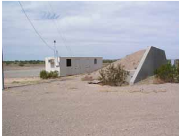
Control Room behind berm
