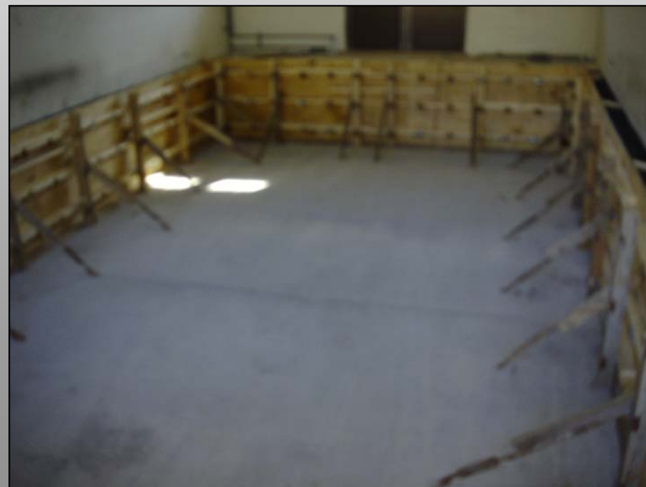
Construction of Containment Pit for Solution Tank
