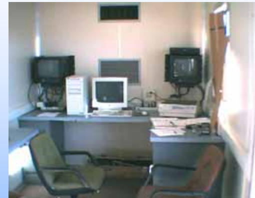
Control building interior
