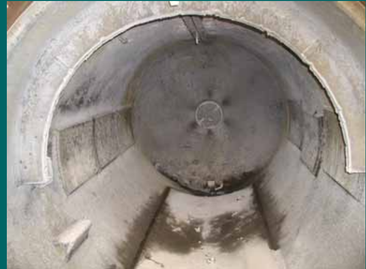
Inside chamber after cleansing shot
