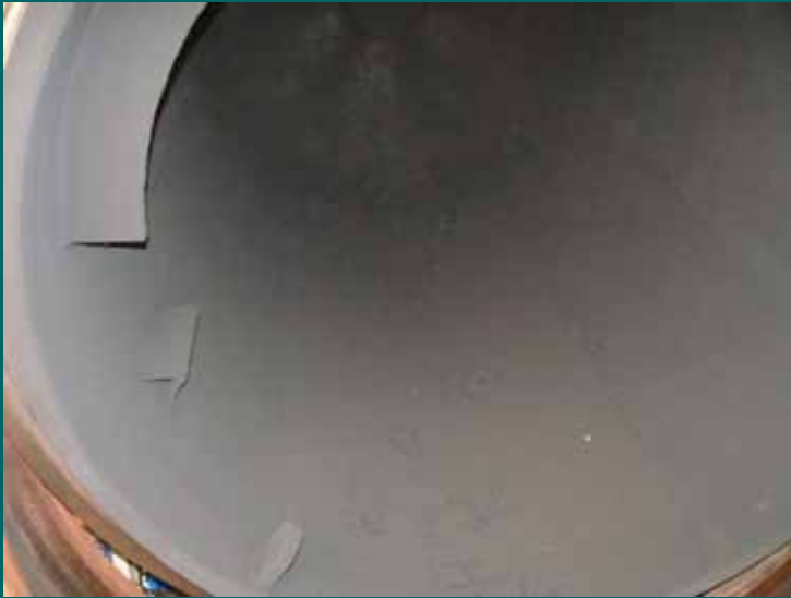
Inside chamber after detonation of bomb and before cleansing shot
