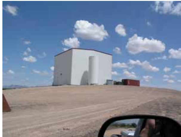
Building, LN2 Tank, Control Room
