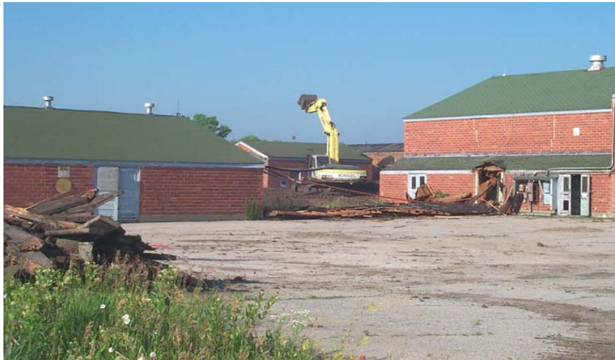
Building Remediation or Demolition Cornhusker Army Ammunition Plant (AAP)
