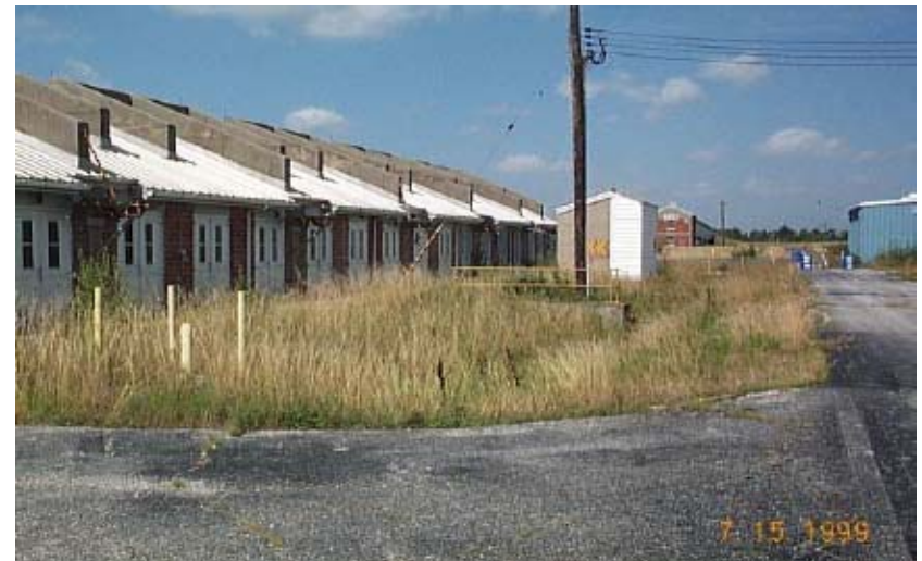
Building Remediation or Demolition Kansas AAP
