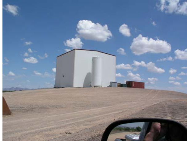
Building, LN2 Tank, Control Room
