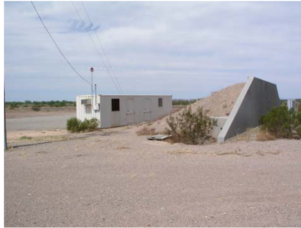
Control Room behind berm
