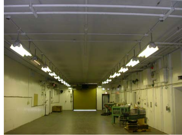
Cryofracture Process Area
