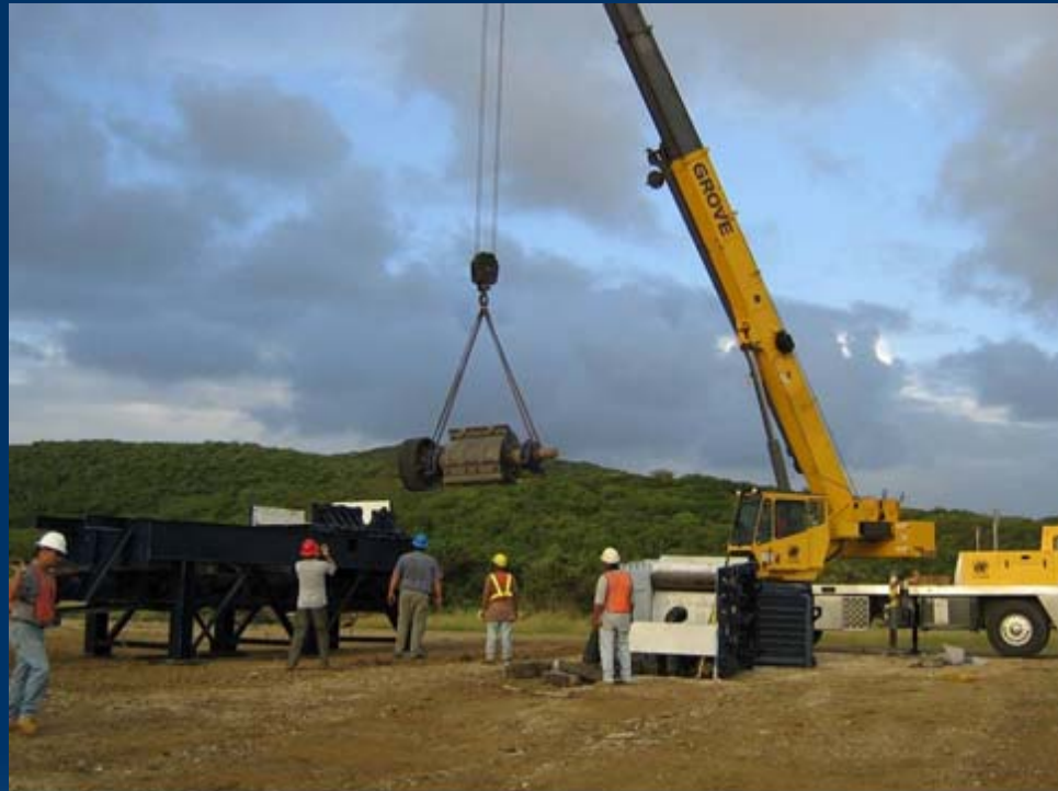
Installation of Impact Crusher using a Crane.
