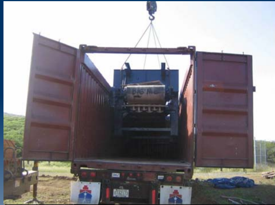
Unloading the Impact Crusher at the CPC
