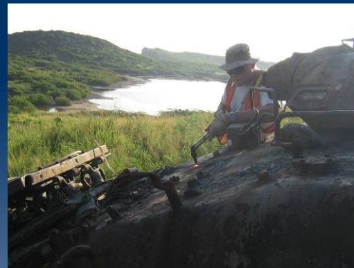
Downsizing target using the Petrogen Torches
