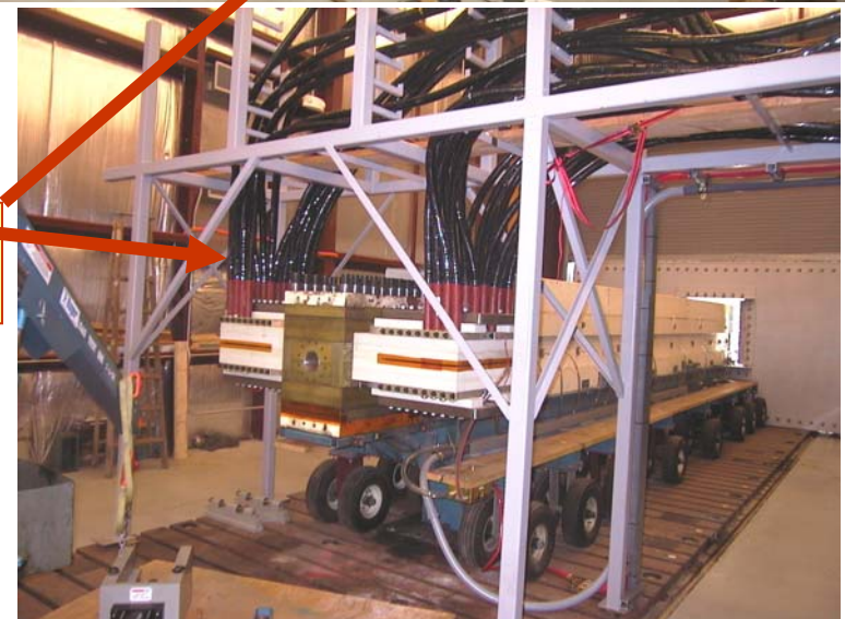
350-MCM Coaxial Cable
