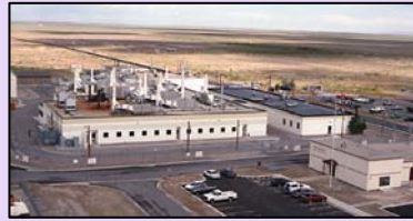
Combined Chemical Test Facility
