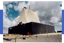
Early Warning Radar
