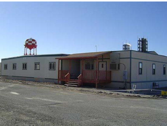
Offices for 45 personnel
