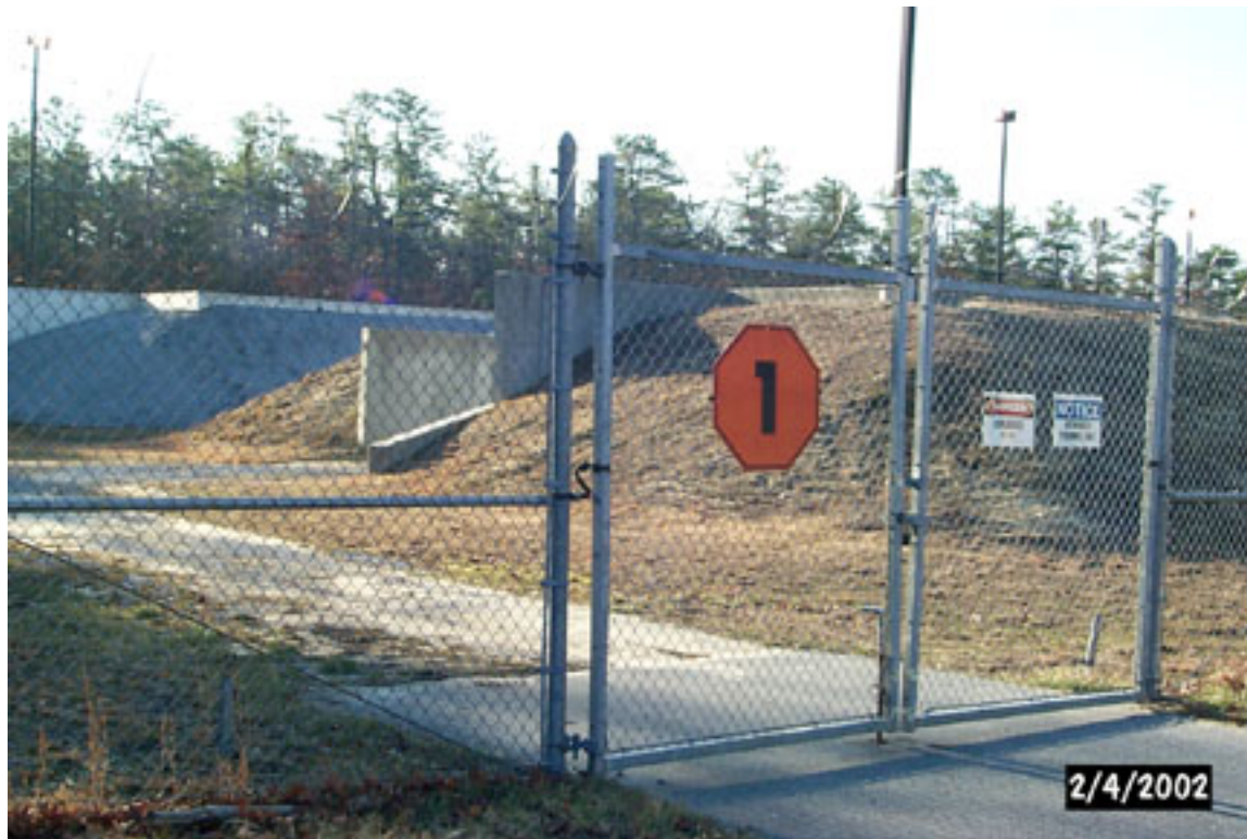
Explosives Storage Bunker
