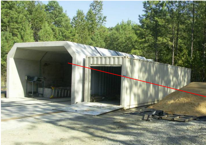
Terminal Back-Stop Construction
