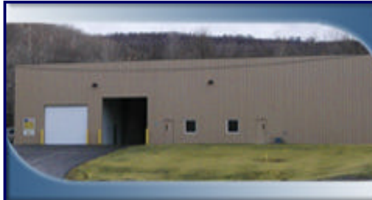
Advanced Manufacturing Laboratory located in Derry, PA
