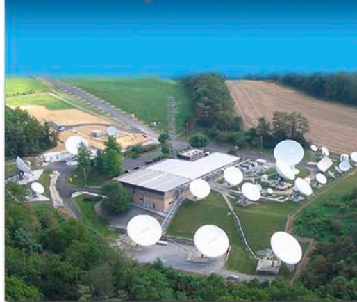
Space and ground satellite communications systems
